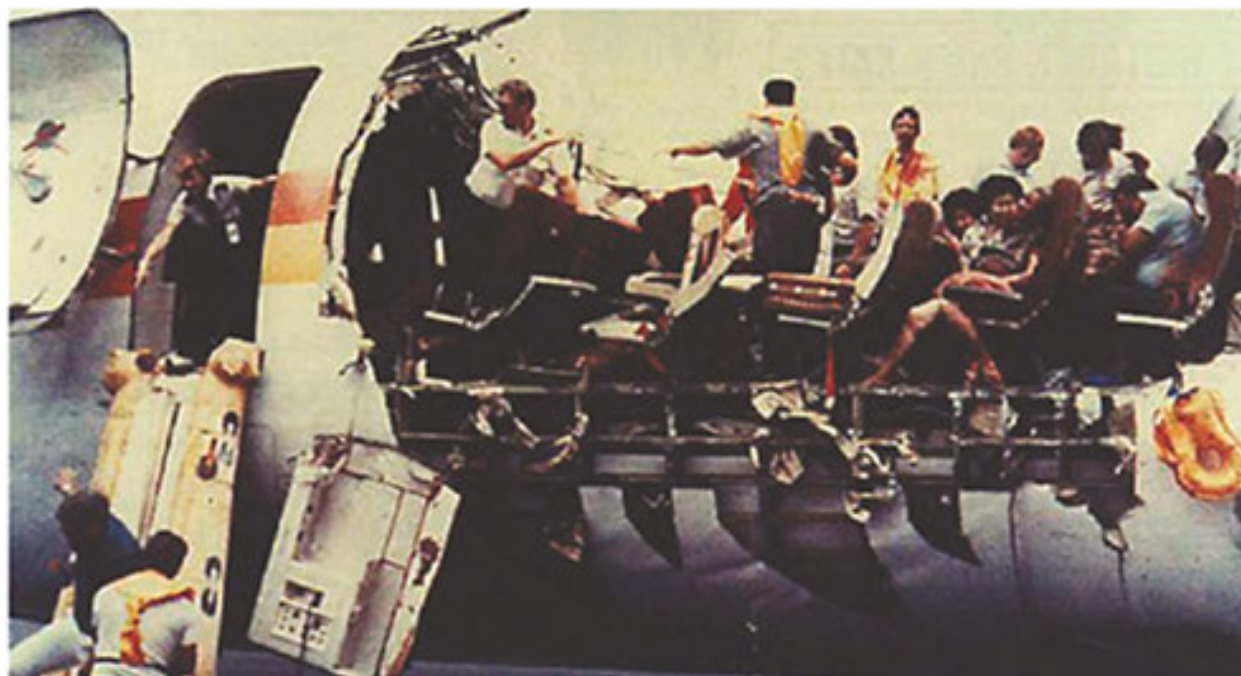
Figure 3. Photography of the flight accident happened at 28th of April 1988 due to corrosion fatigue [24].
