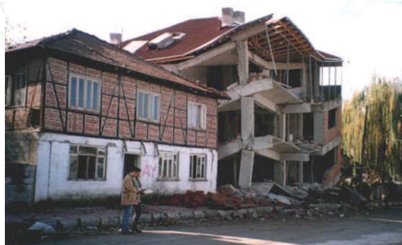
Figure 1. Different damaged conditions of traditional wooden and reinforced concrete buildings after the 1999 Duzce earthquake. Image taken from [6].
