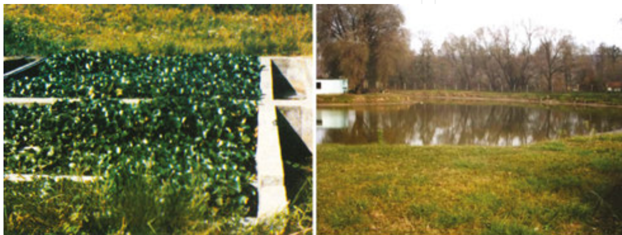
Figure 7. Basin for sanitary hydrophytocultures and basin for sanitary aquacultures on the WWTP Sokobanja.
