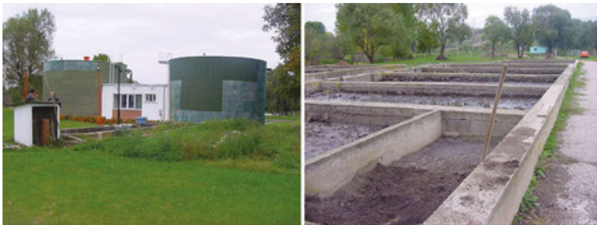
Figure 8. Sludge digester and vermiculture field on the WWTP Sokobanja.
