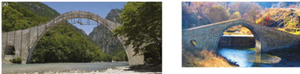
Figure 52. (a) Maintenance works at Plaka Bridge sometime before its collapse from flooding and (b) stone-masonry bridge at Dasilio-Grevena, Greece after being retrofitted.
