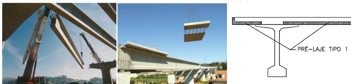
Figure 8. Placement of precast beams and pre-slabs.
