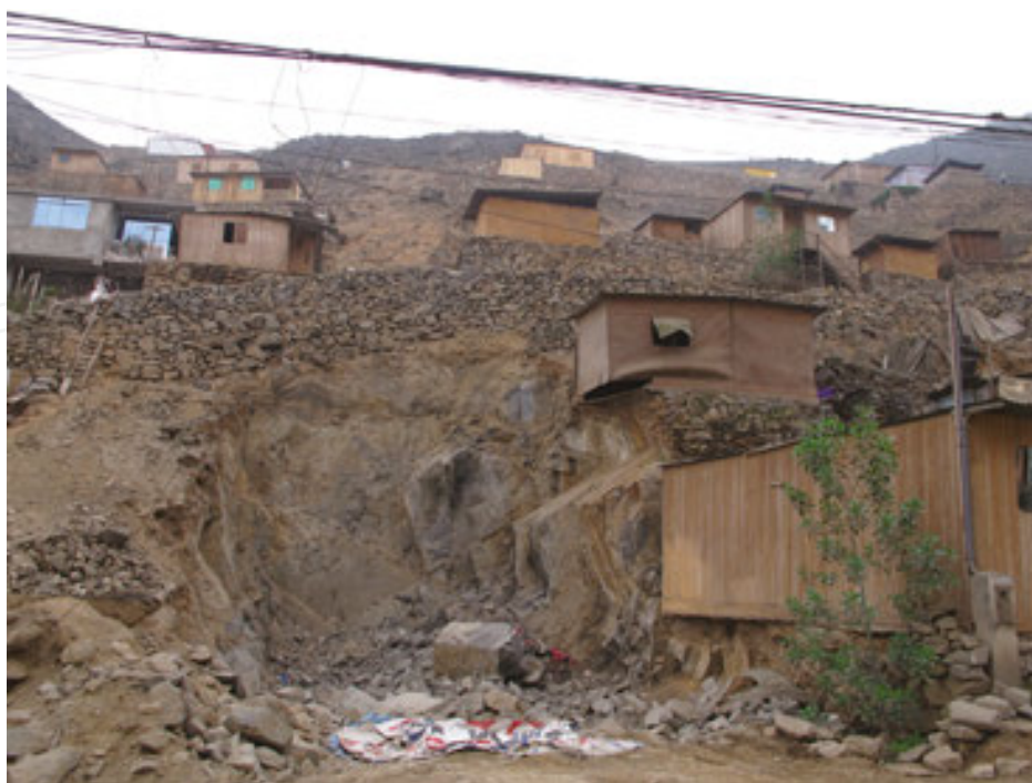
Figure 6. As people flatten the plots to then build their house, they contribute to the instability of the slope and increase the risk for others. Source: Photo by Rita Lambert.
