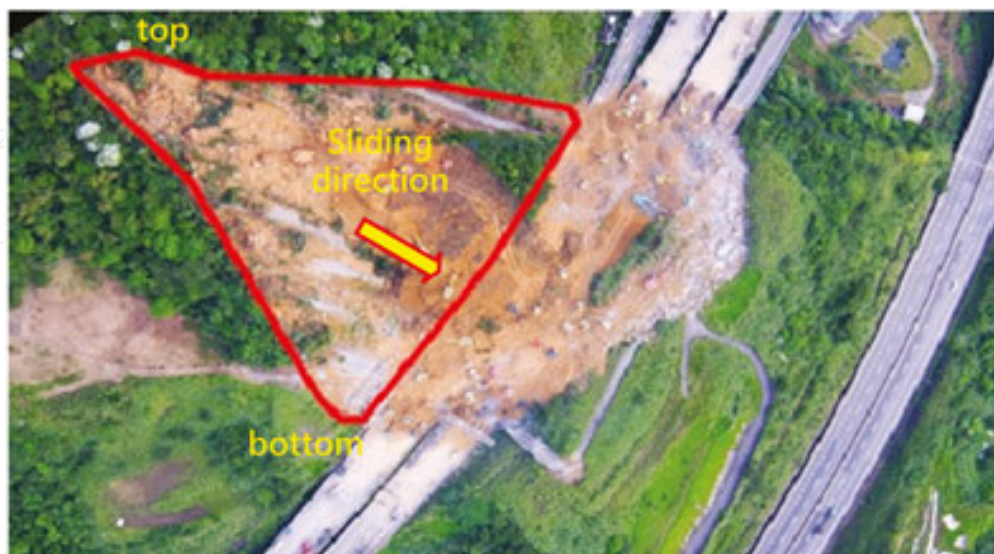
Figure 9. Side boundaries of the landslide and the freeway limits [23].
