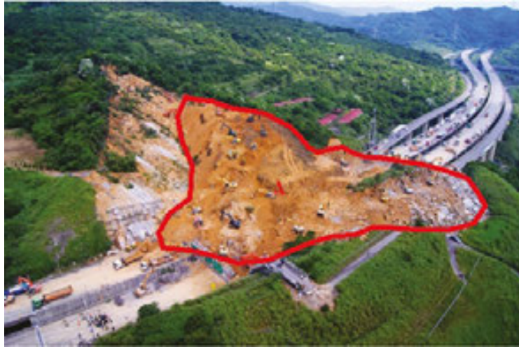
Figure 6. UAV side-view of the landslide taken by a rotary wing UAV owned by Flying Tiger Helicopter and Skyline Dynamics Co., Ltd.
