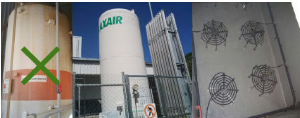
Figure 15. Dosing system for sewage.
