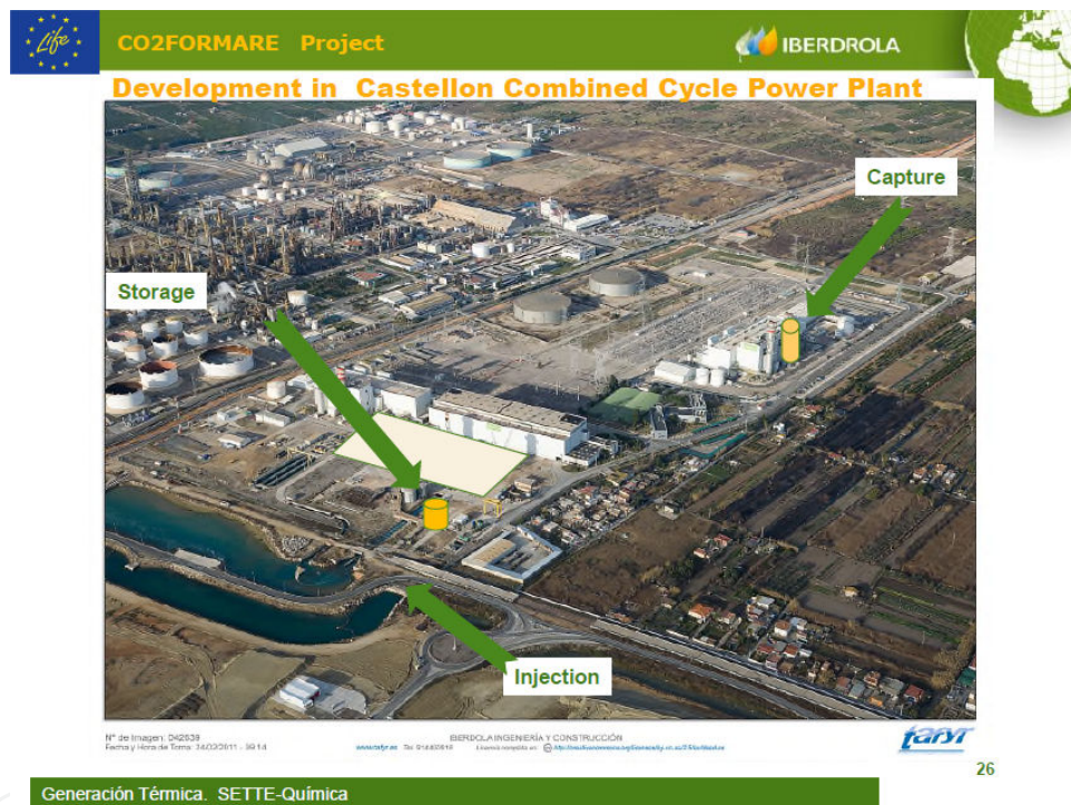
Figure 23. Castellon Power Plant. Courtesy: Iberdrola.
