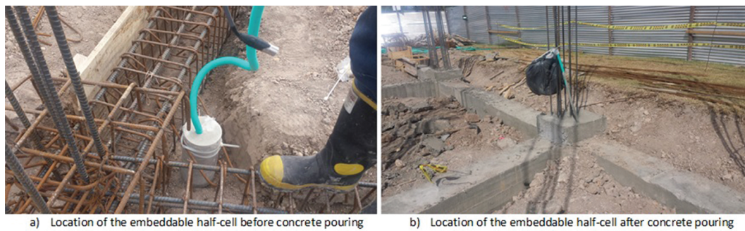
Figure 9. Installation of the embeddable half-cell.
