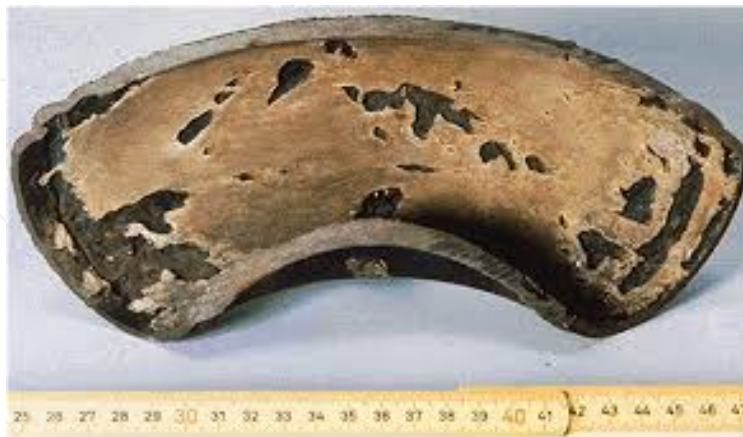
Figure 7. Erosion Corrosion on Inner Surface of an Elbow Pipe [22].
