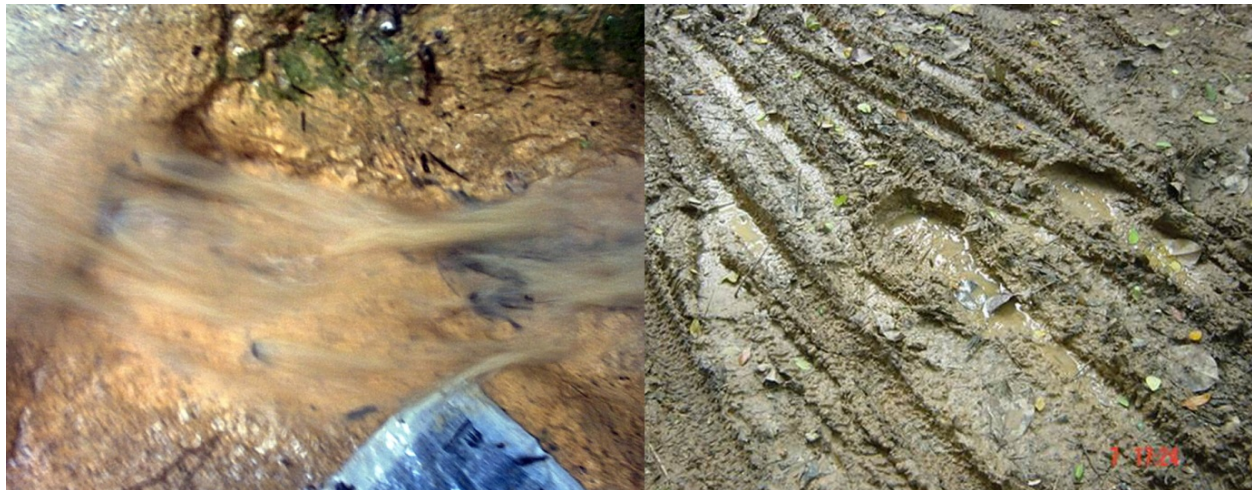
Figure 15. Trail conditions during heavy storms, with bike marks and surface wash (Note the surface wash on the left)
