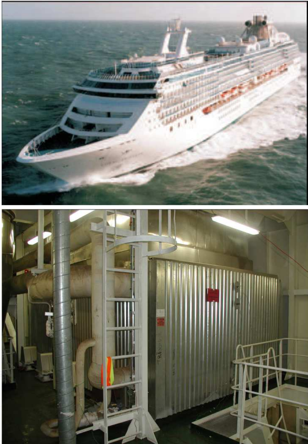
Figure 10. Coral Princess at sea and boiler installed on ship [63]
