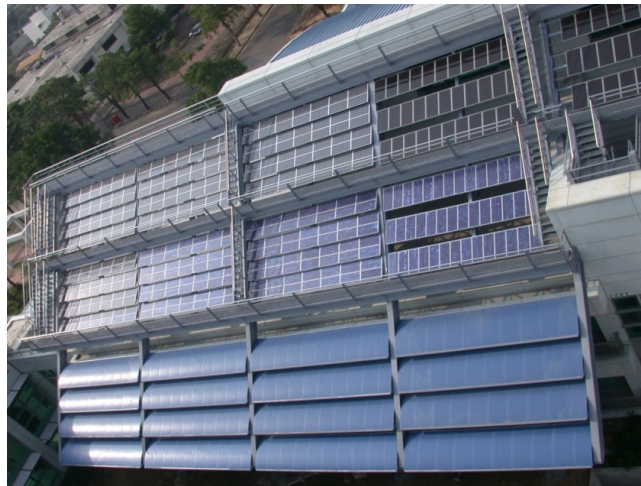
Figure 4. Final Photo of experimental installations in test filed
