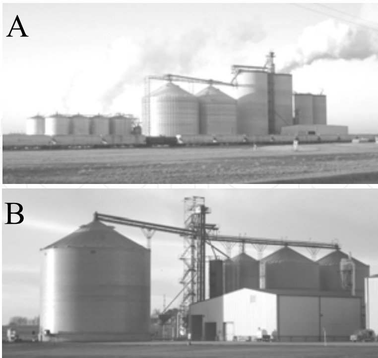
Fig. 3. U.S. dry grind corn-to-ethanol manufacturing plants. A. 450 \times 10^6 L/y plant. B. 80 \times 10^6 L/y plant (Photos courtesy of Rosentrater).
