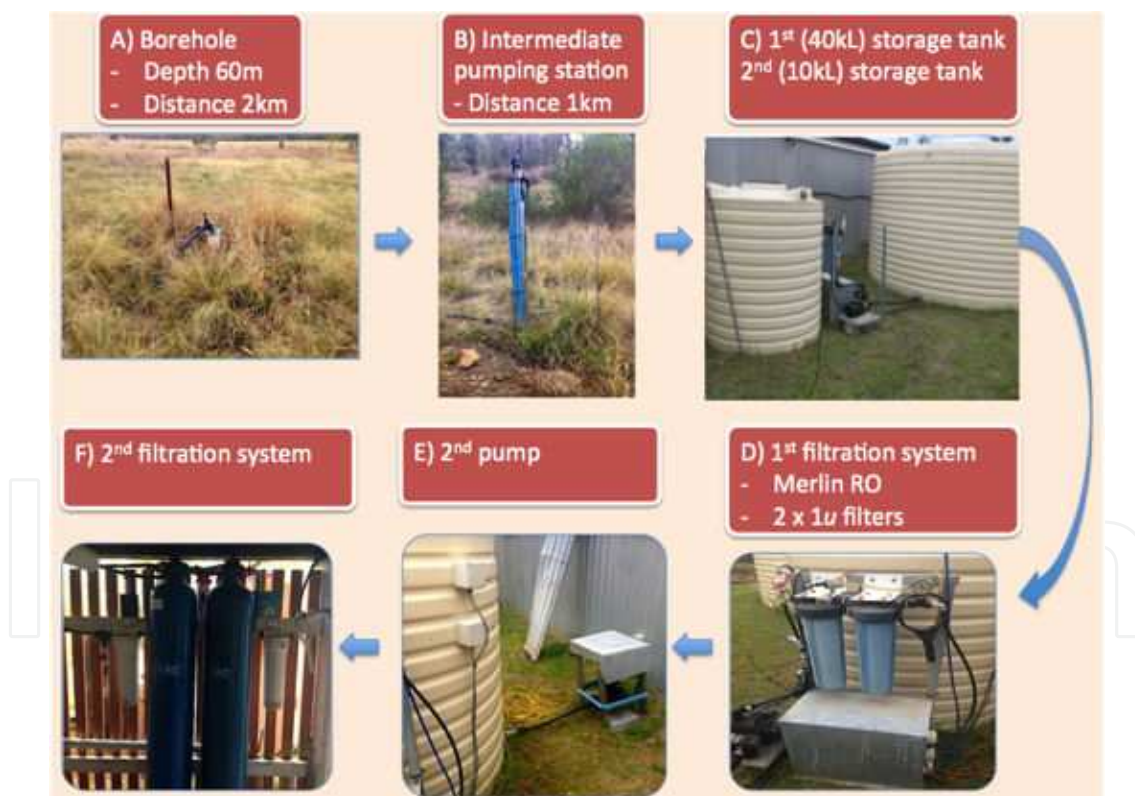
Figure 12. An Example of a rural home water treatment setup: (A) The borehole is approximately 2 km from the patient's residence and is determined by the geology of the area. (B) An intermediate pumping station operated using air pressure. (C) Storage tanks are continually replenished from the bore to ensure an uninterrupted water supply. (D) A basic pre filtration cartridge filter (located in the silver casing) and two micron filters pre treat the water (E) A second pump located approximately 100m from the patients residence (F) A second set of micron filters and carbon tanks. This is located underneath the patients home and feeds directly to dialysis machine inside the bedroom.
