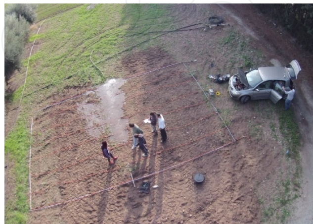
Figure 4. Leakage event in Mandria as observed from UAV
