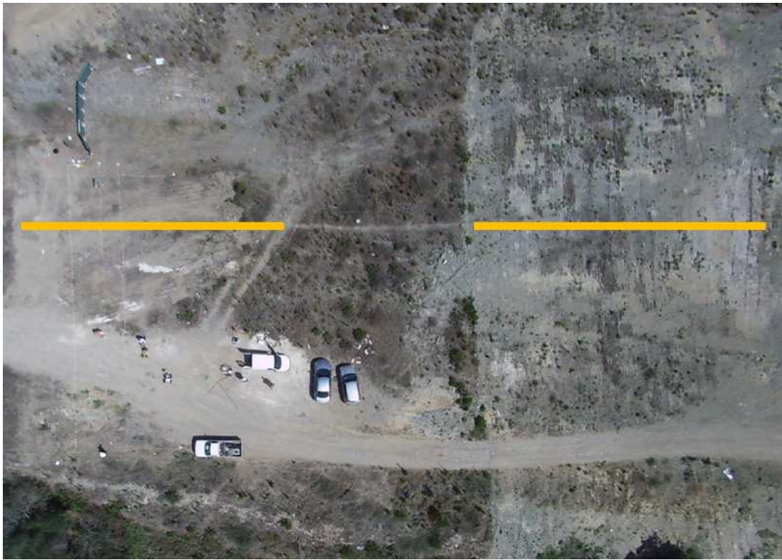
Figure 5. Lakatameia underground pipeline as observed from UAV
