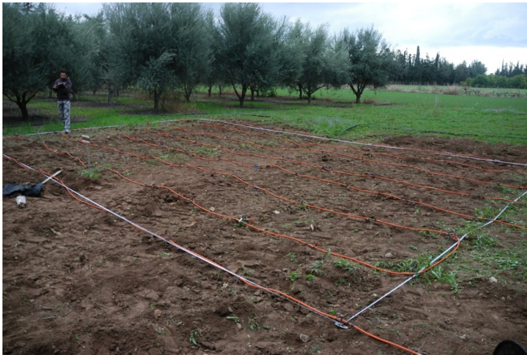
Figure 1. Area of interest. A pipeline was buried at a depth of approximately 1 meter.
