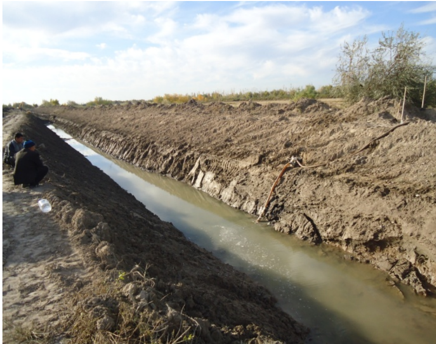
Figure 5. Gravity flow of water in the plastic lined channel
