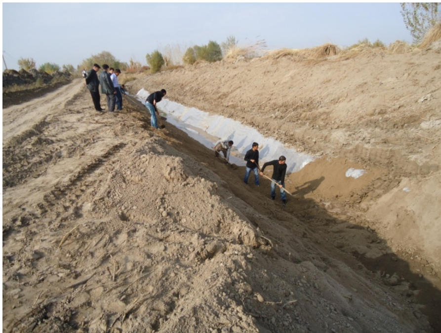
Figure 4. Covering of plastic with compacted soil
