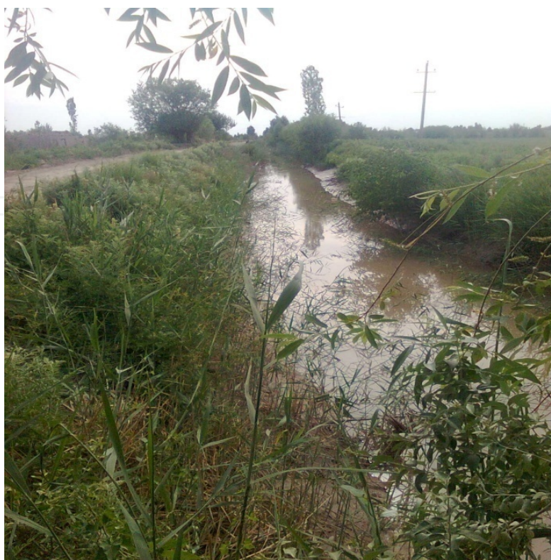
Figure 1. Appearance of the channel prior to plastic lining
