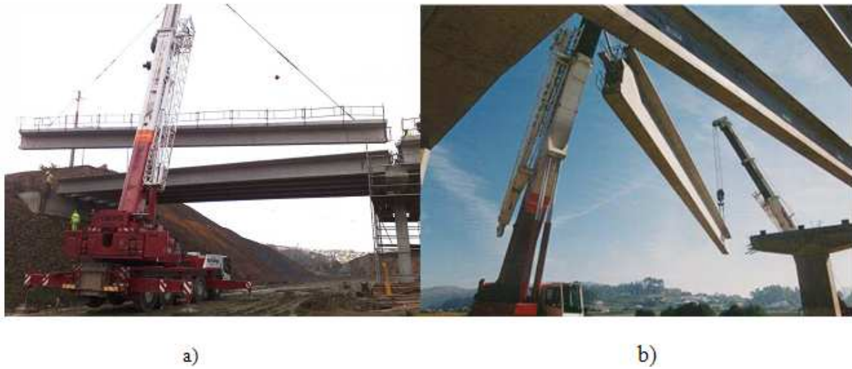
Figure 6. Placing of precast beams on the pillars (Leonhardt, 1982).
