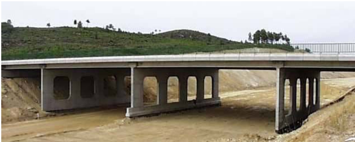
Figure 4. Overpass on A23 performed with prefabrication (Juntas, 2013)
