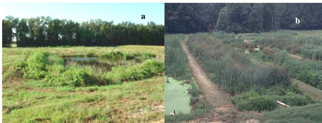
Figure 6. a. Settling basin. Picture courtesy of Auburn University; b. Constructed wetlands in Mississippi (Tucker 2009) (BMP No. 6 2002).
