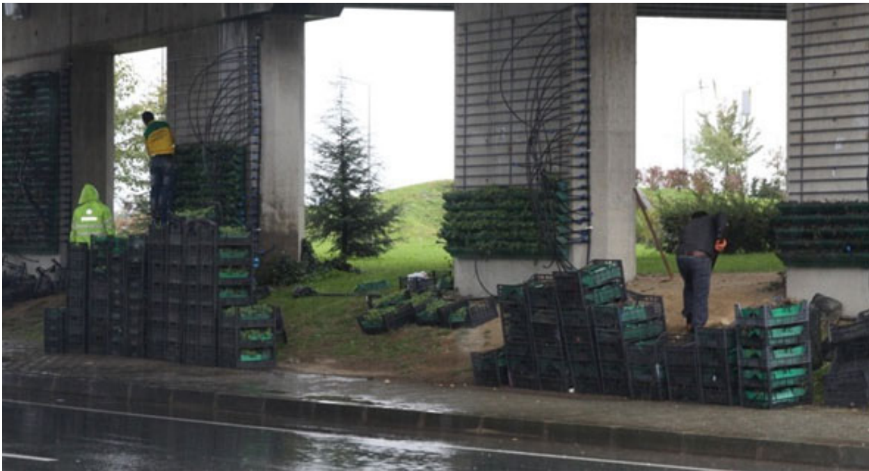
Figure 42. Viaduct pillars from Rize ( http://www.zaman53.com 2013).
