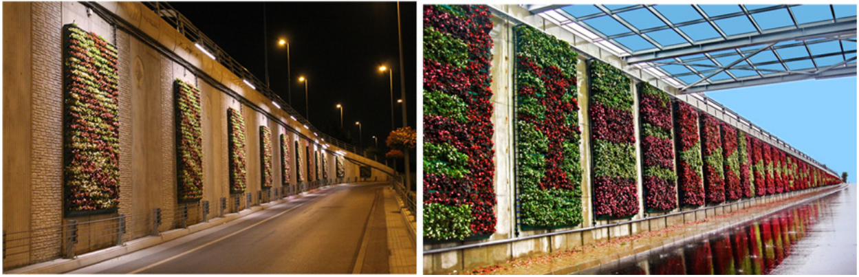
Figure 41. İstanbul airport roadside (left), Antalya airport roadside (right) ( http://www.aktasplant.com 2013).
