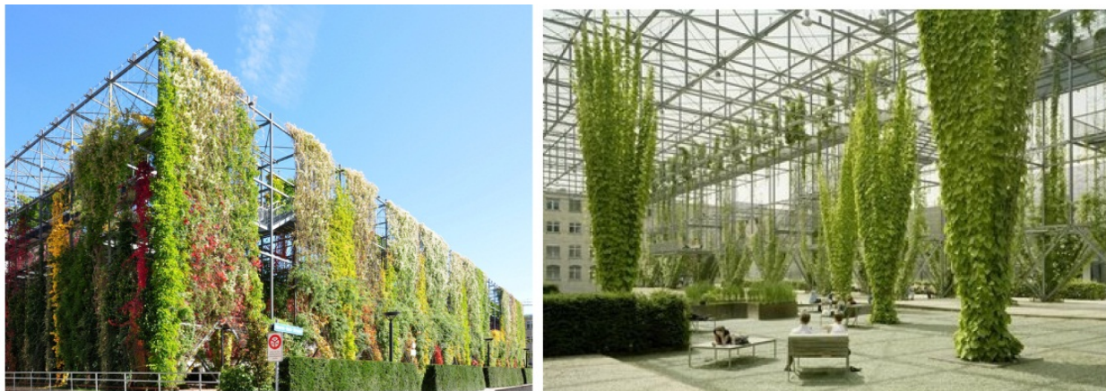
Figure 6. Grid and Wire-Rope Net Systems, MFO Park Switzerland ( http://commons.wikimedia.org 2013, http://christianbarnardblog.blogspot.com 2013).
