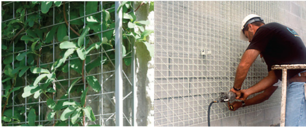
Figure 13. Modular trellis panel system (Green roofs organization 2008).
