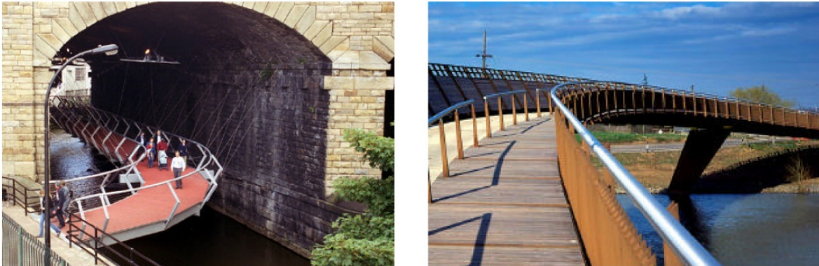
Figure 23. An examples of innovative designs, Dark River Irvel in Manchester (APEM and Environment Agency, 2010)
