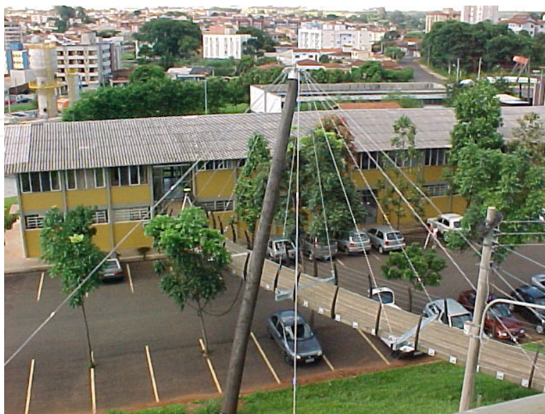
Figure 9. Cable- Stayed wood footbridge in Sao Carlos Engineering School, USP
