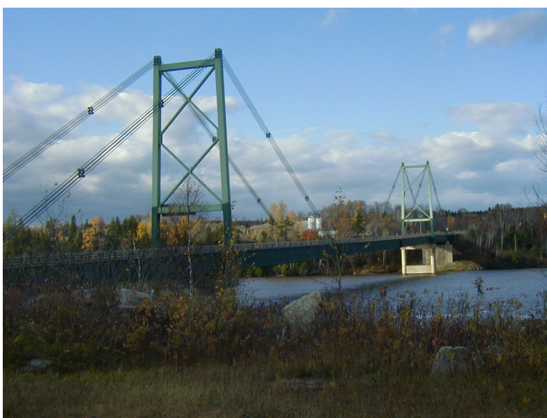
Figure 10. Hawkshaw Cable-Stayed Bridge, New Brunswick, Canada
