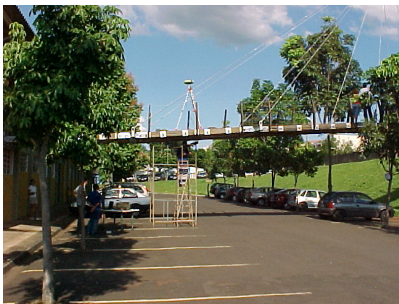
Figure 13. The GPS receiver and transducer of displacement installed in a footbridge
