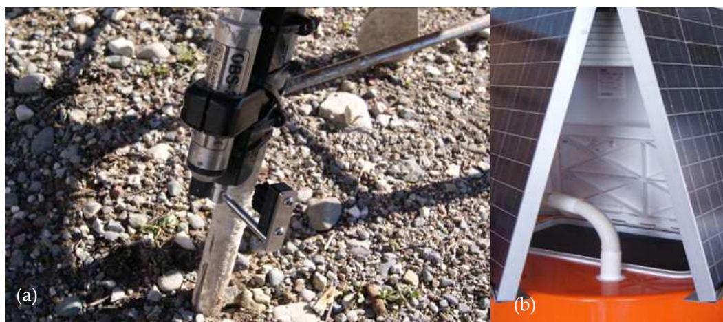
Figure 9. a) Turbidity optical sensor and (b) humidity sensor located on a floating buoy deployed in Asprokremmos Dam.
