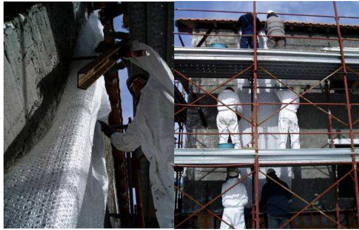
Figure 20. Application of technical textiles containing POF on a masonry building at the Eucentre in Pavia, Italy.
