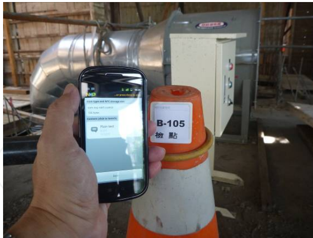
Figure 7. Splayed the staff updated the inspection information in jobsite checkpoint location
