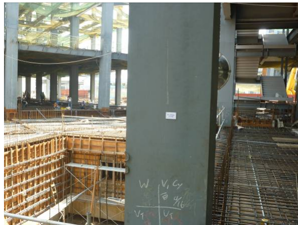
Figure 3. Displayed the safety checkpoint location attached UHF RFID tag in the case study. (A)
