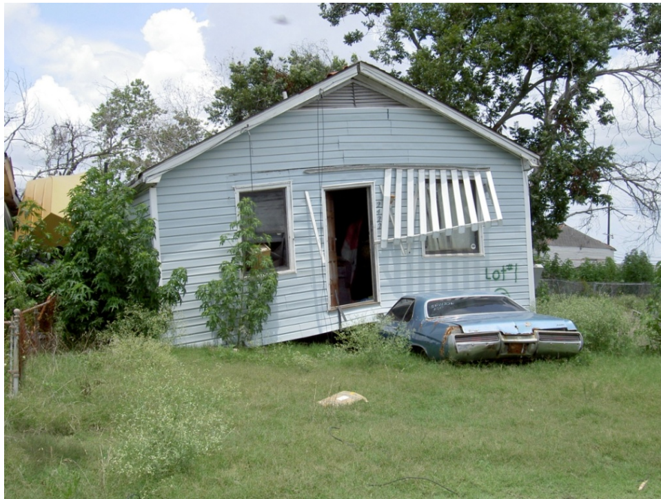
Figure 5. Katrina damage in Lower 9th Ward
