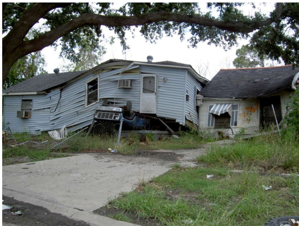
Figure 4. Katrina damage in Lower 9th Ward
