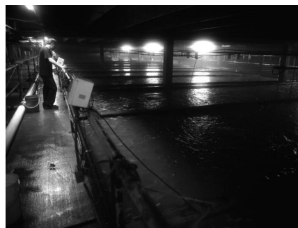
Figure 1. Commercial-scale tilapia grow-out systems at Blue Ridge Aquaculture. The grow-out units are to the right of the catwalk and sedimentation basins to the left. Photograph courtesy of Blue Ridge Aquaculture.
