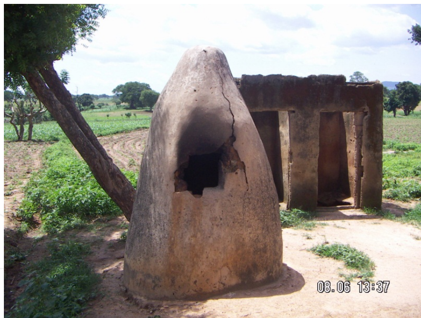
Figure 3. Locally developed incinerator using mud blocks
