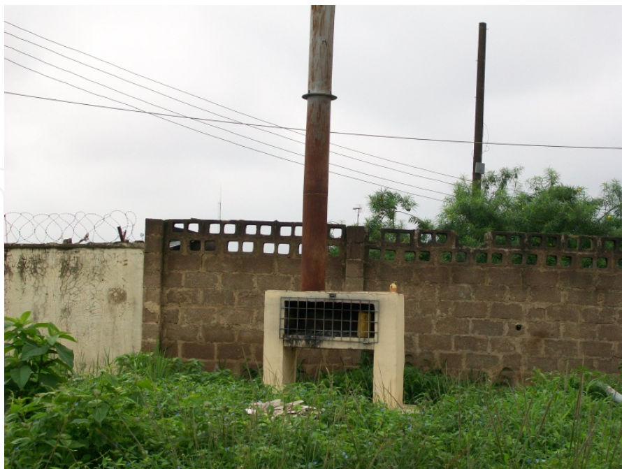
Figure 1. Locally developed incinerator using concrete
