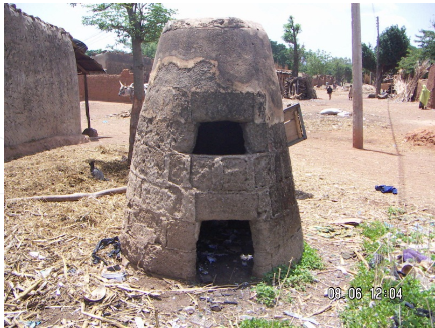
Figure 2. Locally developed incinerator using sandcrete
