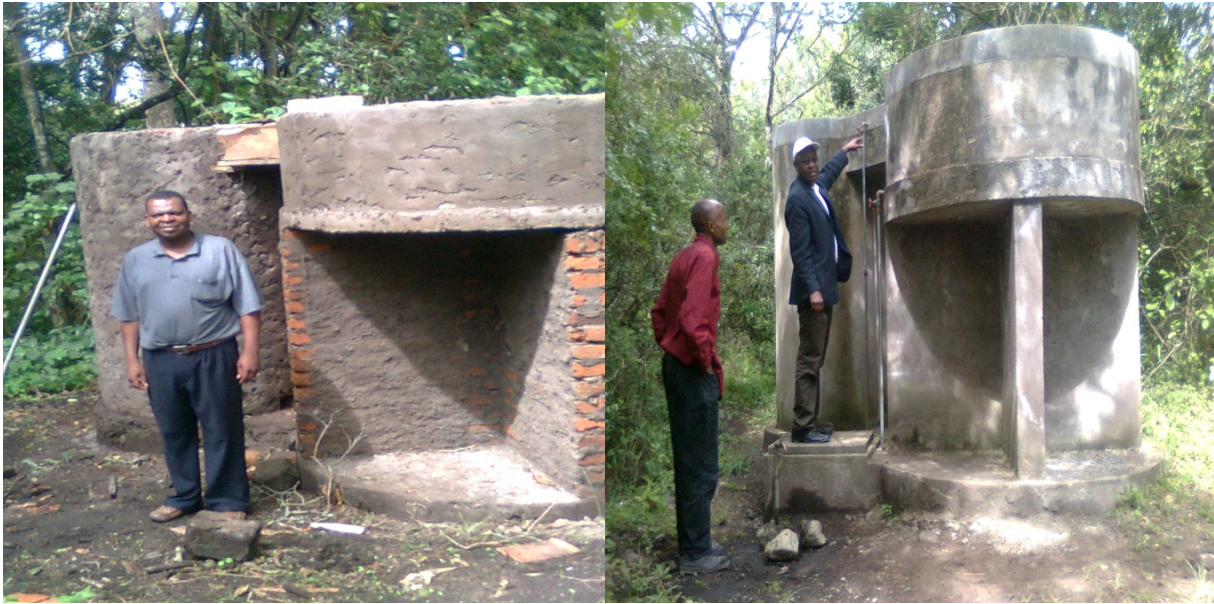
Figure 13. Incomplete and completed community defluoridation unit designed by Ngurdoto Defluoridation research station
