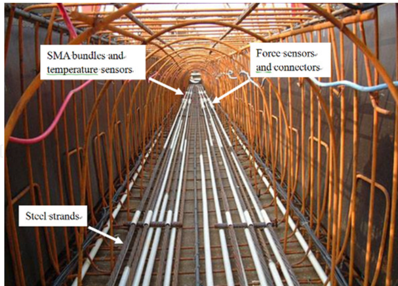
Figure 32. Framework of steel reinforcement with stretched SMA bundles
