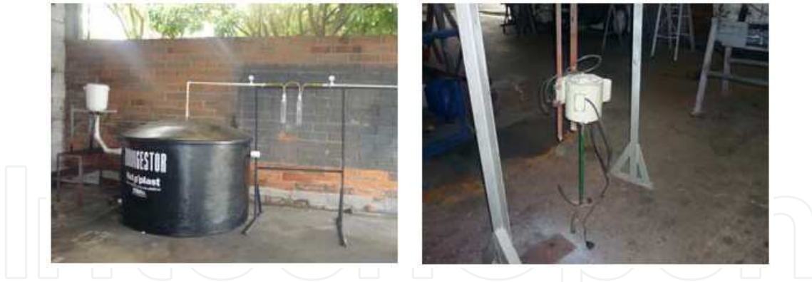
Figure 3. Installation of bioreactor and equipment to trituration
