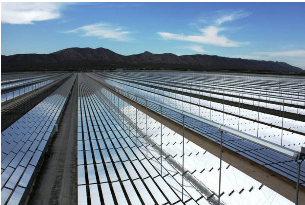
Figure 6. Linear Fresnel reflectors in the power plant Thermosolar Power Plant (PE2) in Spain [46].
