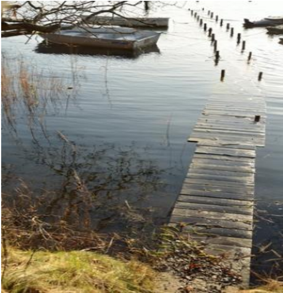
Figure 7. Flooded dock. Sea levels around the world can be expected to rise by several metres in coming centuries, if global warming carries on. Even if global warming is limited to 2 degrees Celsius, global-mean sea level could continue to rise, reaching between 1.5 and 4 metres above present-day levels by the year 2300, with the best estimate being at 2.7 metres. (Credit: © knuderik / Fotolia)
