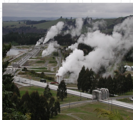
Figure 8. Steam pipelines towards the Wairakei Geothermal Power Station [24]
