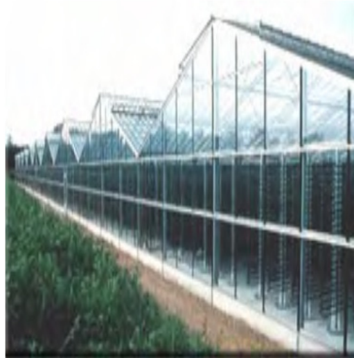
Figure 14. Glass tube photobioreactor (700 m 3 ) producing Chlorella biomass (Klötze, Germany)
