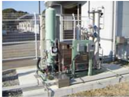
Figure 12. The adsorptive, isolated methane concentrating device
