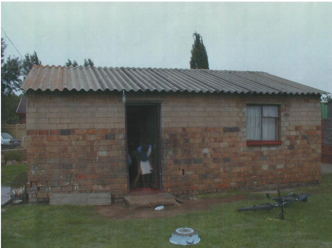
Figure 2. Typical house in Soweto near Johannesburg built circa 1960 with an asbestos cement roof. (Courtesy of Professor JI Phillips).
