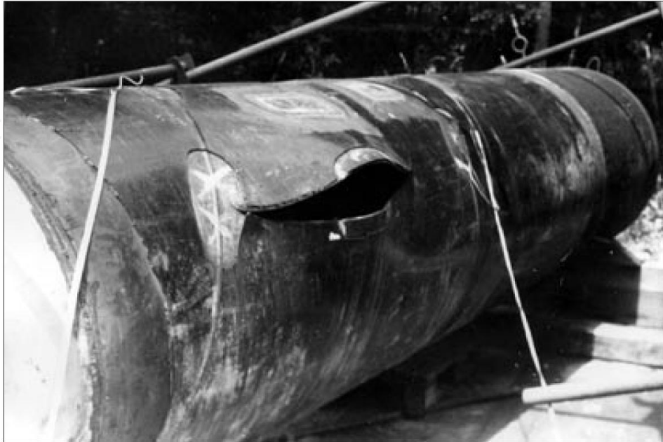
Figure 16. Burst initiated on slit B with a fatigue crack
