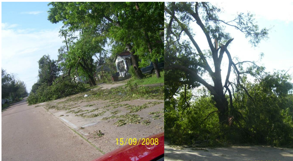
Figure 10. Tree damage and debris along Hardy Road, ca. 2 km from the tower site.
