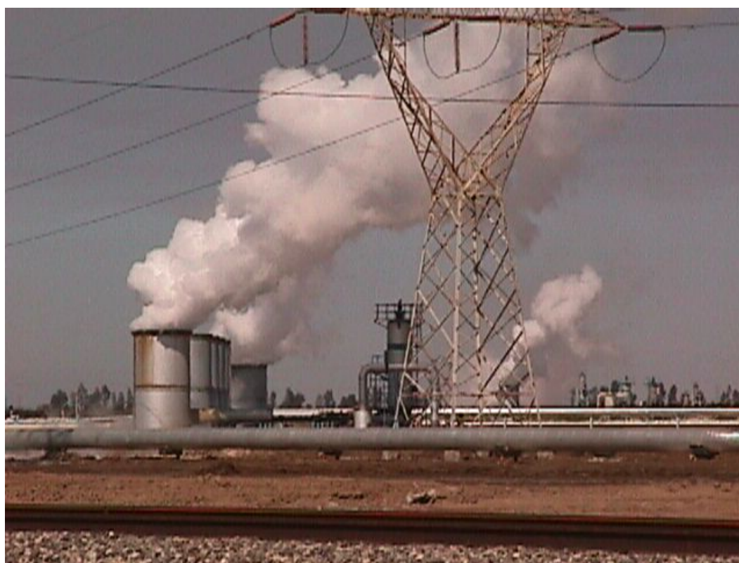
Figure 16. A humid corrosive environment in a geothermal field caused by steam and gases emission.
