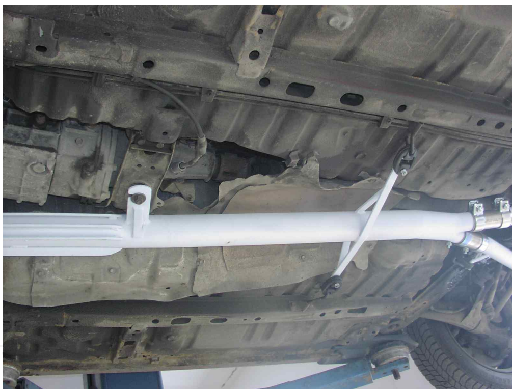
Figure 13. Corrosion on carbon steel exhaust pipes coated with aluminum.
