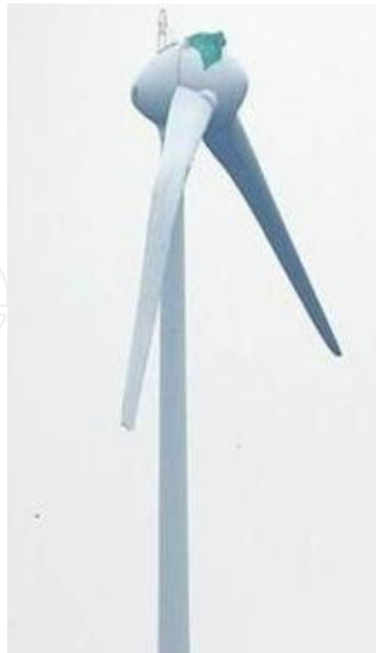
Figure 3. Typical blade failure of a three-bladed, 2 MW wind turbine
