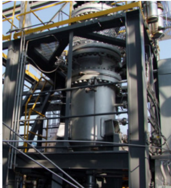
Figure 3. Pilot-scale coal gasifier of membrane wall, top-feeding, slagging type (max. 21 bar)
