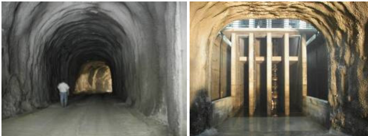
Figure 5. Socorridos storage tank: inlet tunnel (on the left) and centrifugal pump (on the right)
