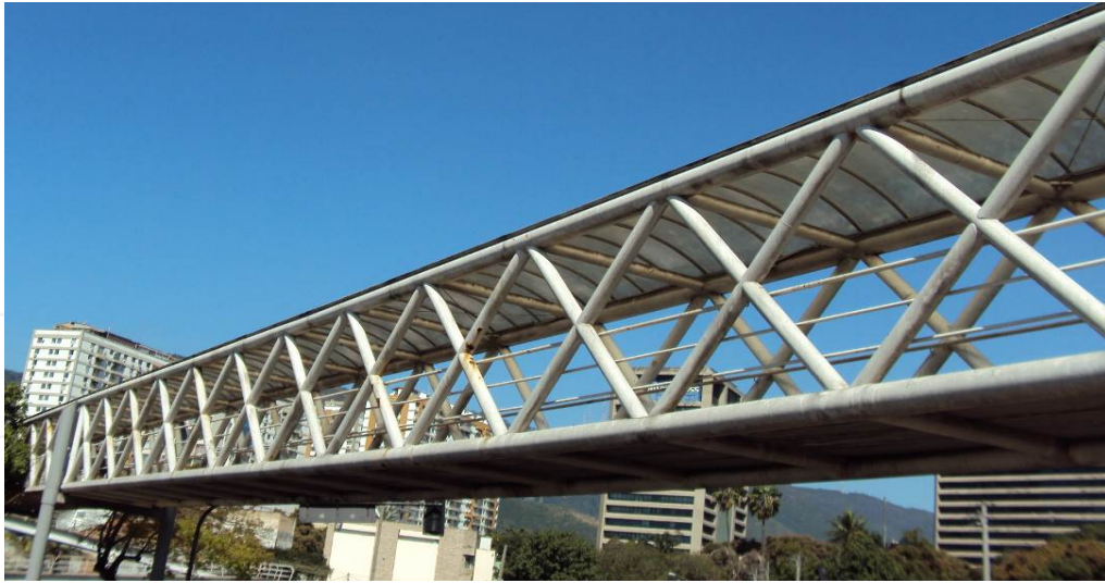
Figure 7. Investigated steel-concrete composite tubular footbridge.
