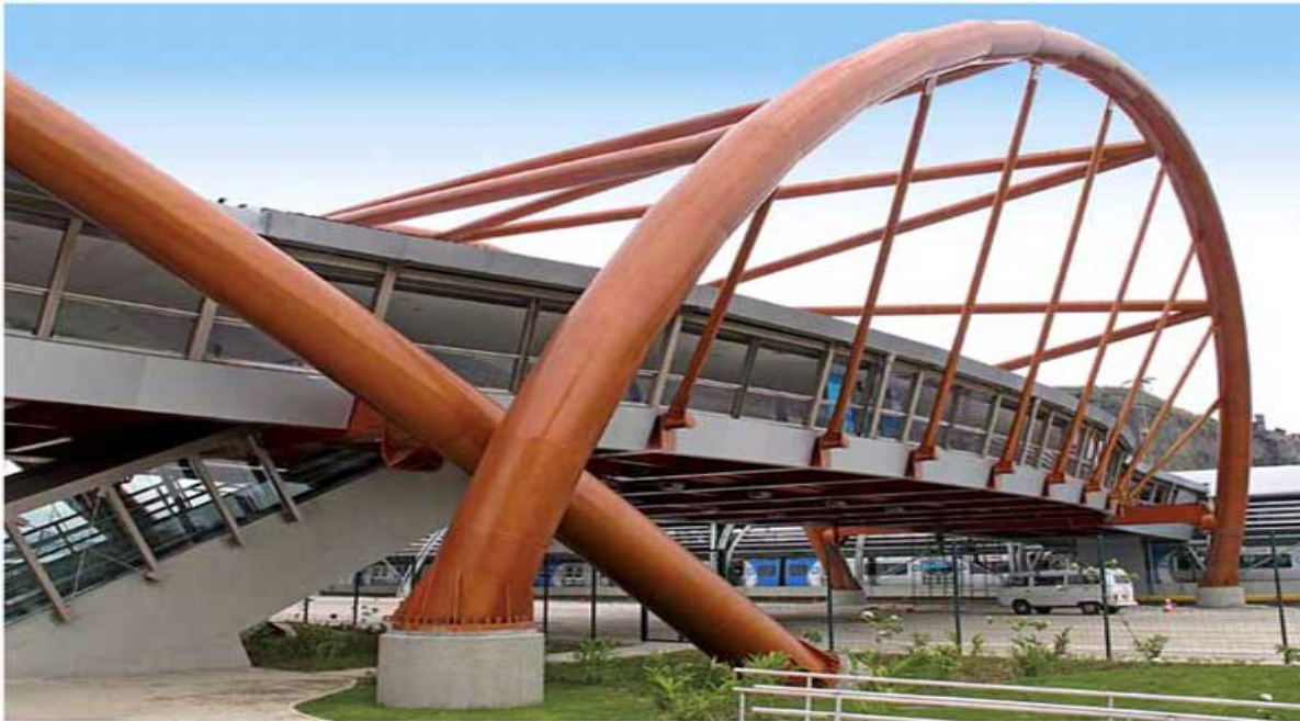
Figure 1. Example of a tubular steel pedestrian footbridge in Rio de Janeiro/RJ, Brazil.
