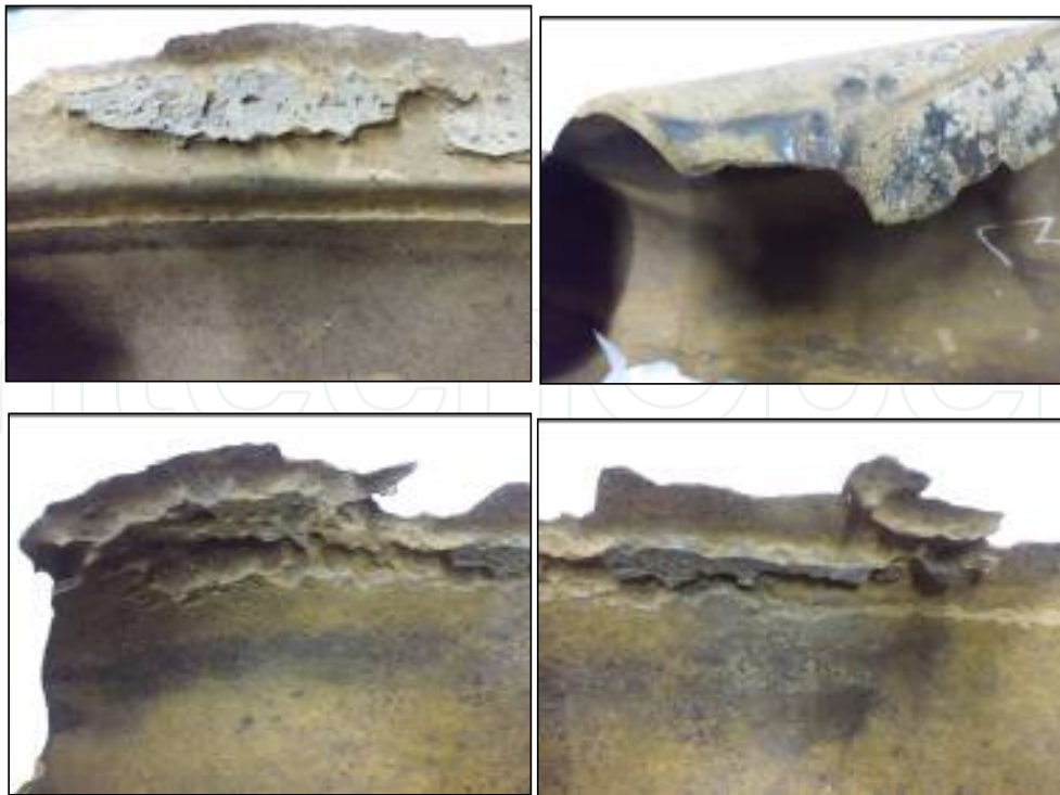
Figure 7. Wall thinning and pits at 5 – 7 o'clock position of downstream part.
