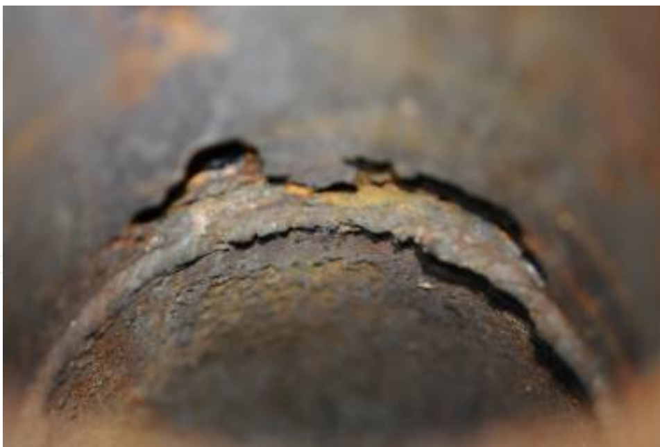
Figure 15. An excessive overfill and severe surface degradation beside overfill at 6 o'clock position.
