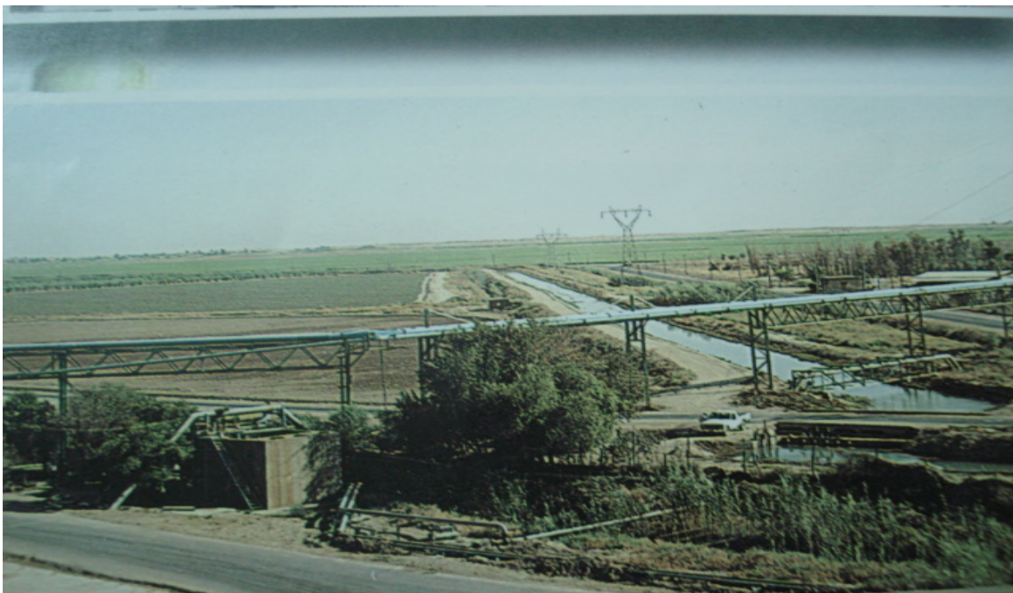
Figure 5. Transported the Bagasse through pipe from the sugarcane factory to the paper factory
