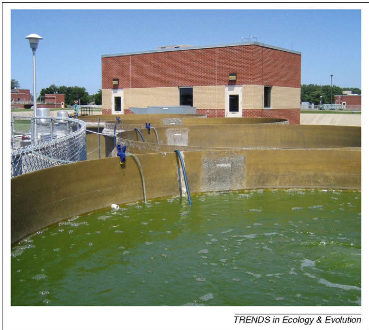
Figure 2. Dense algal growth in four pilot-scale tank bioreactors fed by treated wastewater from the Lawrence, Kansas (USA) wastewater treatment plant (photo by B. Sturm). Each fiberglass bioreactor has an operating volume of ten cubic meters of water, and is operated as an air-mixed, flow-through vessel. Nutrient-rich wastewater inflows are pumped in through the clear plastic hose (blue clamp), and water outflow occurs through the white plastic pipe shown at the waterline. These bioreactors are intended to be operated year-round, as the temperature of the inflowing wastewater is consistently ca. 10 - 8°C.
