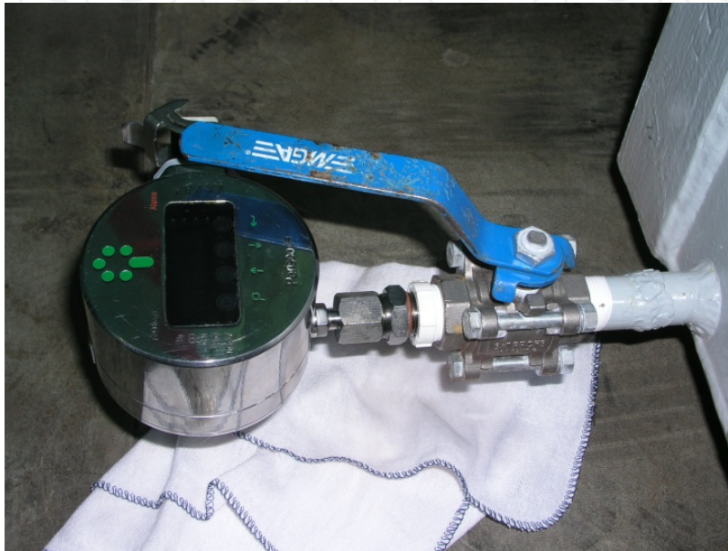
Figure 5. Gas analysis sensor installed in the experimental tank.
