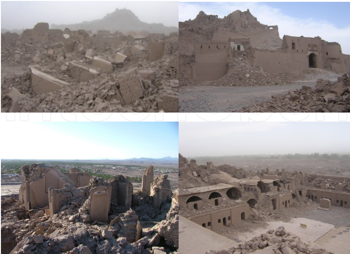
Figure 1. Citadel of Bam after earthquake in 2003
