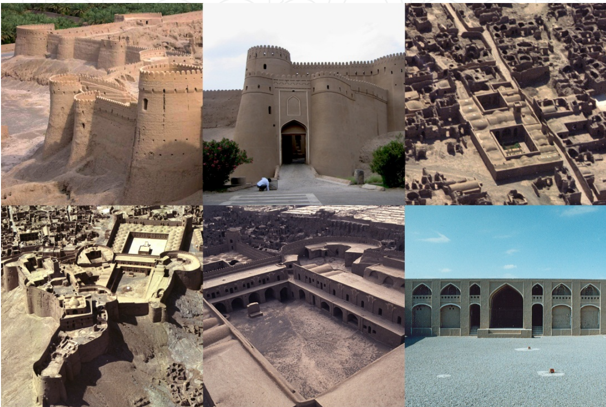
Figure 2. Architecture of citadel of Bam and its different types of buildings. Photographic credits: ICHHTO (top left, center, bottom center, and right) and NCC (top right and bottom left)
