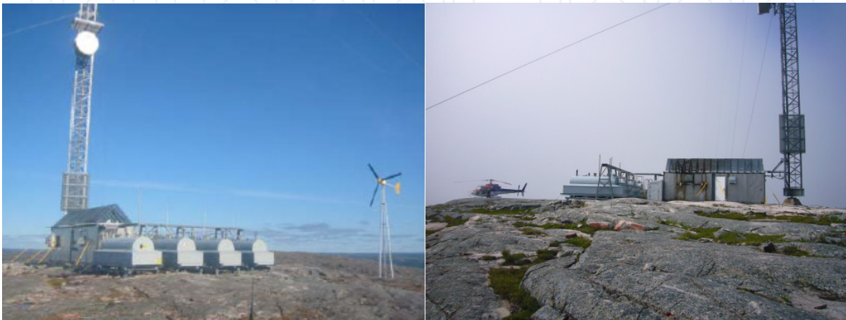
Figure 19. Telecom station of Bell-Canada at Kuujjuarapik [37]
